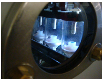
Three phase visible position of contacts.
