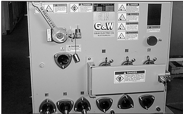
Switch with front mounted fusing.
