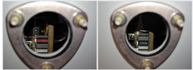
Position indicators provide contact position indication through viewing windows.
