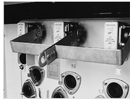
Three phase interrupter operating handle
