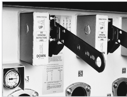
Single phase interrupter operating handles
