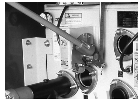
Load break operating handle
