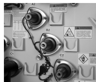
600A voltage sensing bushings
