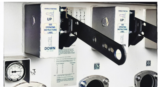
Single phase interrupter operating handles.
