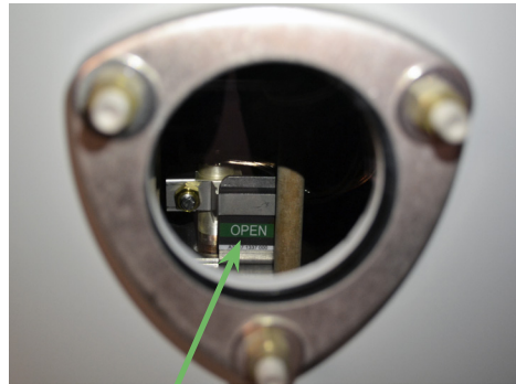
Position indicators provide visible verification of contact position through viewing windows.
