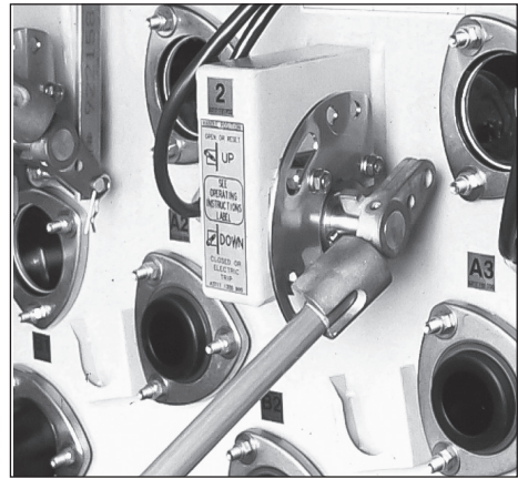
Three phase interrupter operating handle for manual three phase operation and reset.
