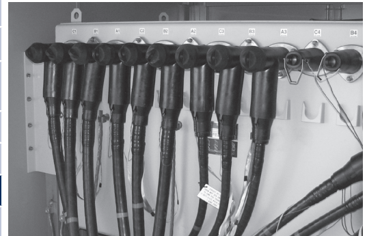
Back view of a padmount PNI-43L with rotary style load break operator.
