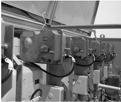
Motor actuators (below) can be added for remote operation.
