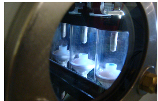
Load break switch visible break
