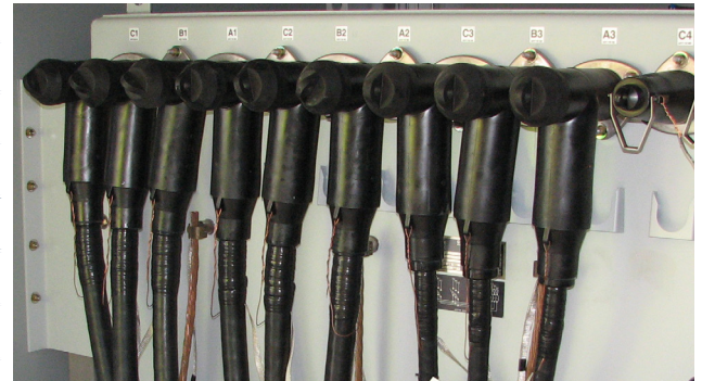
Cable entrances are located on the back of the switch.
