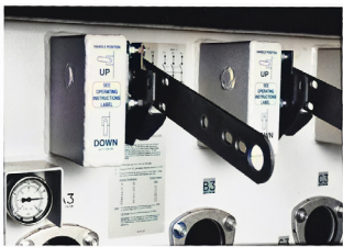
Single phase interrupter operating handles.
